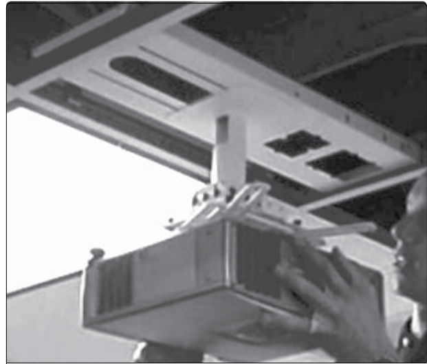
2f Slide and lock the projector onto the adjuster plate
